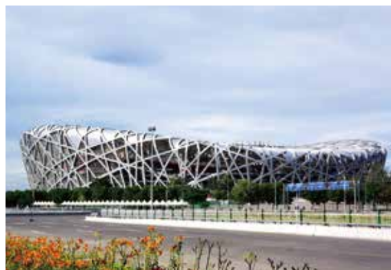
Bird's Nest Stadium project in Beijing
