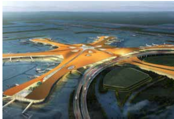
Daxing International Airport project
